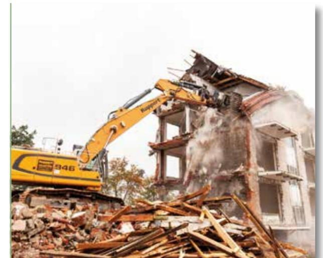
A digger completing the works after selective dismantling
